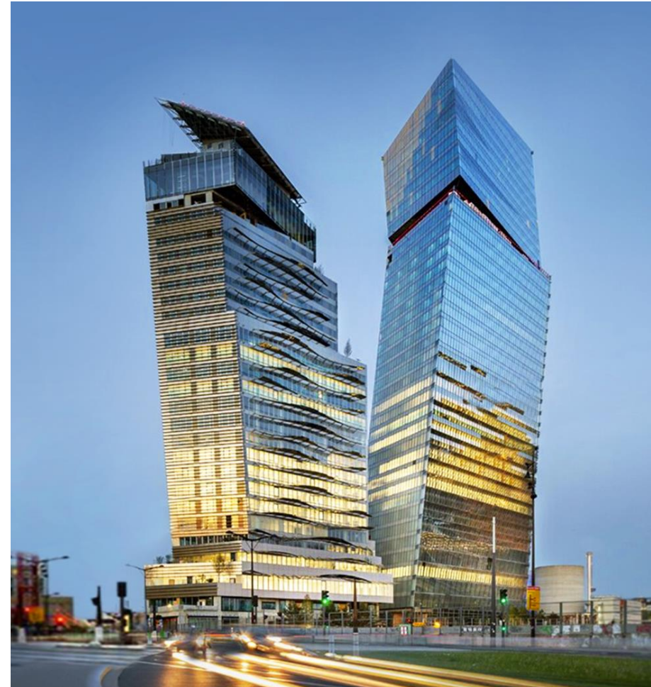
Duo Towers, Paris, France Built with Vertua Concrete, part of our Vertua family of sustainable products Picture by Jad Sylla Photography
